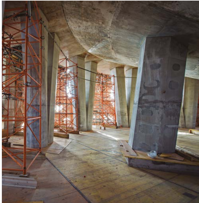
The support columns for the tower of Jesus Christ, as they pass through the lower part of the Crossing Room. They are exposed concrete.
