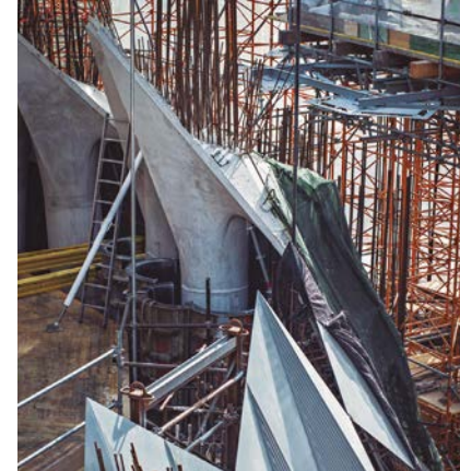
Columns and capitals in white concrete in the Crossing Room. The columns were poured on site using polyester moulds, and the columns were prefabricated using polyester moulds on the Temple grounds and then lifted into place with a crane.
