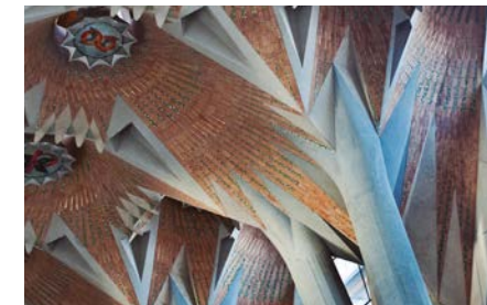
Trunk and branches of a tree and a column meeting the vault.
