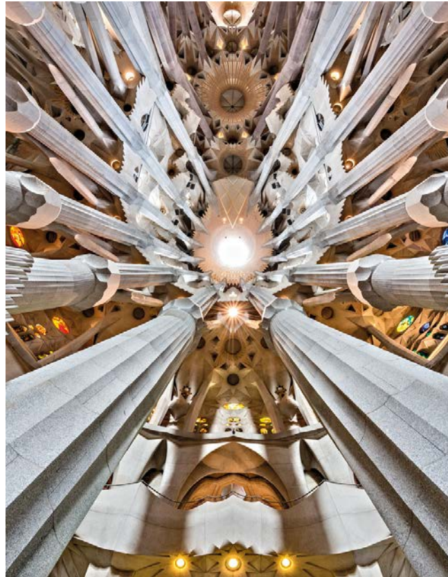
Overhead view of the great hyperboloid covering the apse.
