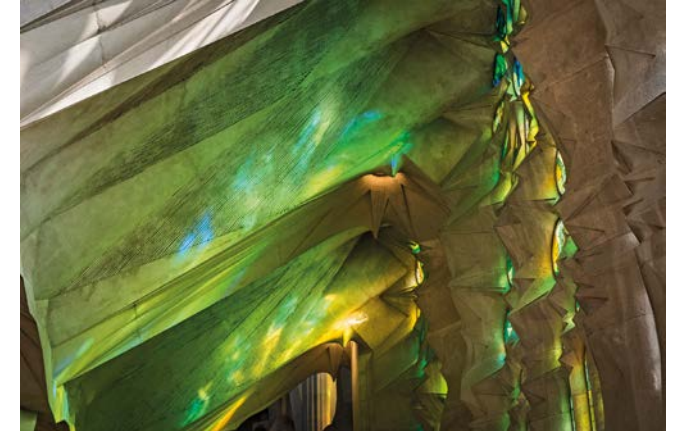
Choir vaults, built using prefabricated concrete pieces and concrete poured on site.
