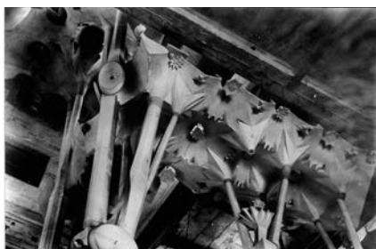
Model of the nave vaults by Gaudí.
