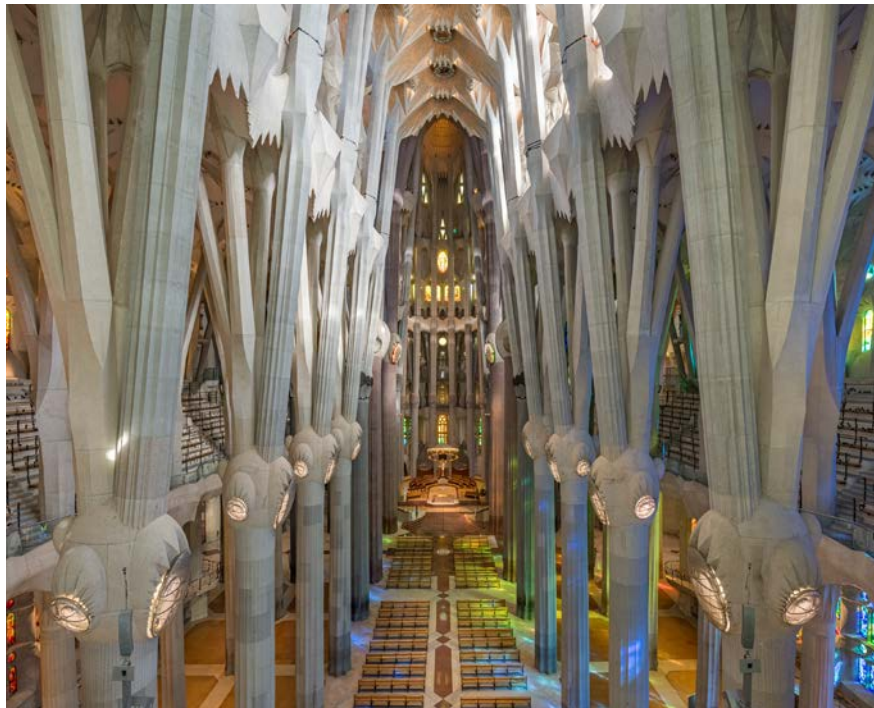
From the knot, the columns branch out at different levels to support the Temple vaults (top).
