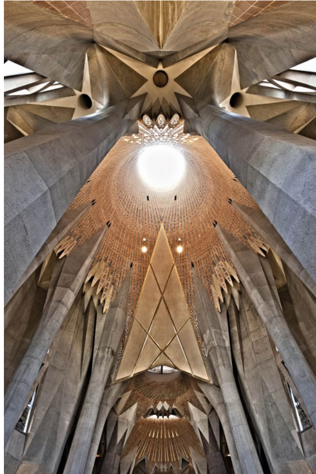
The bright hyperboloid vault on the apse.
