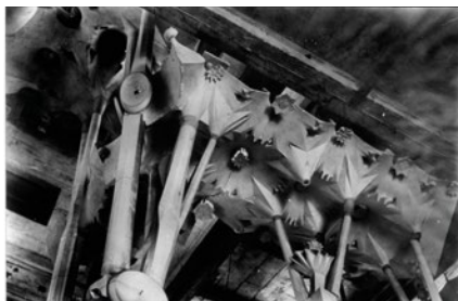
Model of the nave vaults by Gaudí.
